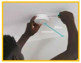
All smoke alarms need to be replaced **EVERY TEN YEARS**. Install smoke alarms with a 10 year long-life battery.
